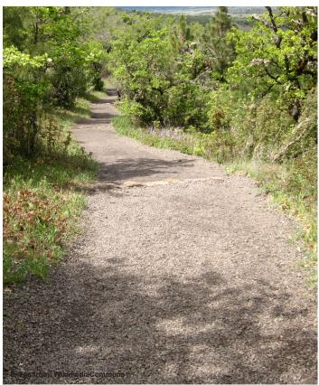
Compacted aggregate path in a nature center
