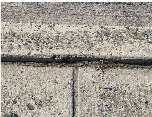
Photo 1 - Before Concrete Lifting
