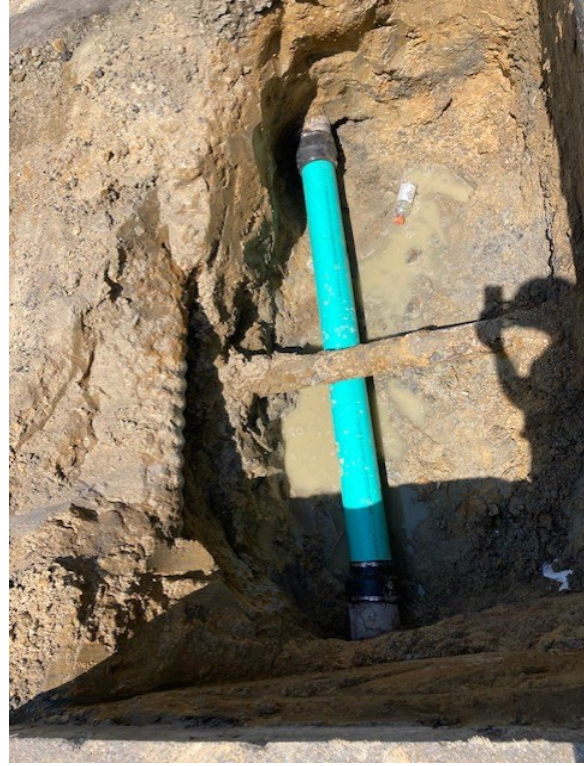
Sewer Lateral Repair West Pine Street
