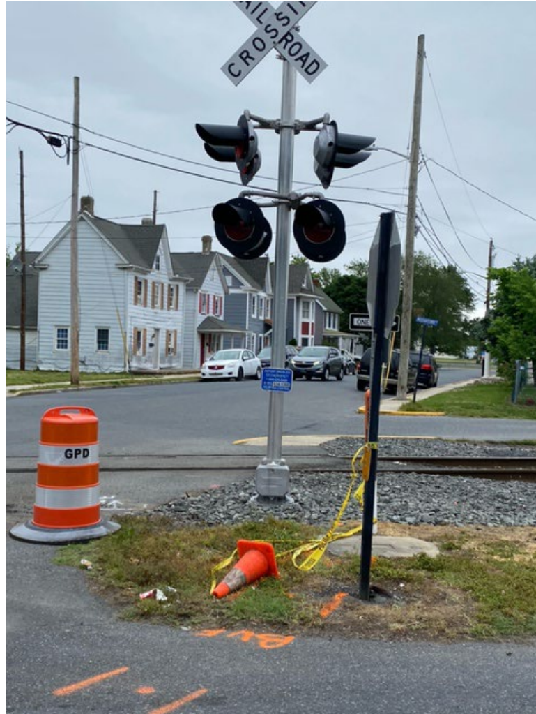
Replaced Railroad Crossing Warning Lights East Pine Street at South Railroad Avenue
