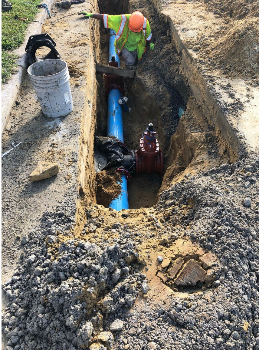
East Market Street Water Main Replacement
