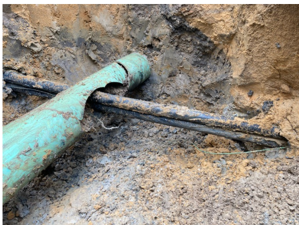
Damaged sewer lateral – East Market Street
