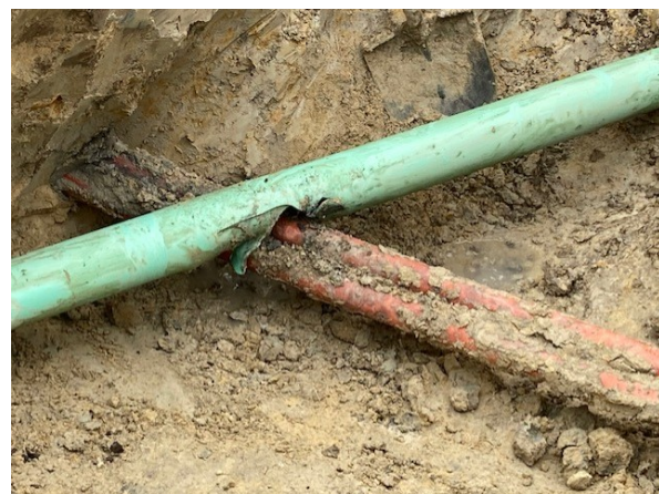
Damaged sewer lateral – East Market Street
