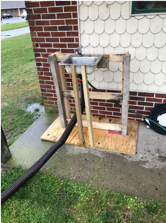
Hand Wash Station
