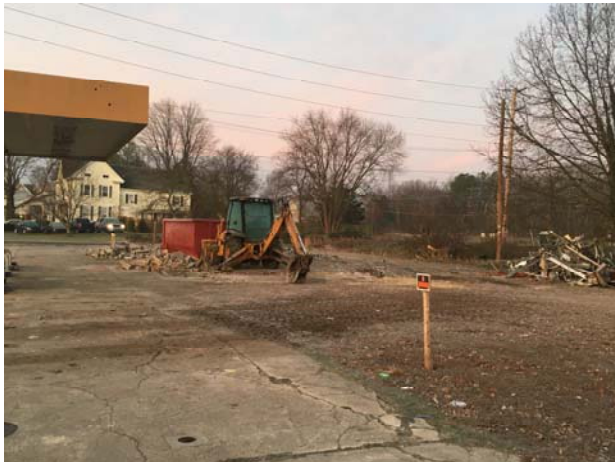
Demolition – East Market Street
