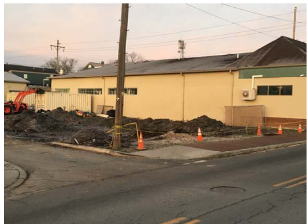
Demolition – Layton Avenue
